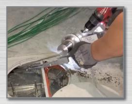
Difficult Walkerduct pulls can be dangerous and delicate. The CP1000 allows you to secure a consistent pressure and steady pull force. Mule tape is easily wound and tailed off the capstan.
