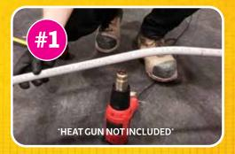
Prep your pipe with a heat source such as heat gun or blanket to make it soft and bendable.
