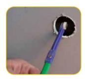
**Step 1**: Find an existing opening or drill a minimum 20mm diameter hole into the surface to create an entry point.
