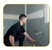
Step 3: Direct The Ferret using the body and feed it through until it reaches the endpoint.
