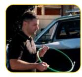
Step 4: Pull The Ferret through the opening. Then coil it up for the next job.
