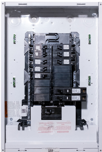
BusGuard with the Panel cover off
