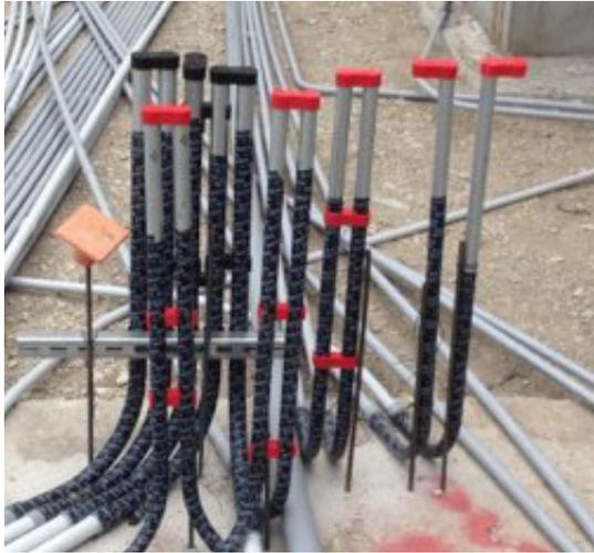
Forget duct tape, tie wires, and wood wedges for 4-square box knockout spacing. Slammers Spacers and caps are the best way to set up and protect your conduit systems to later accept 4-square box knock out.
